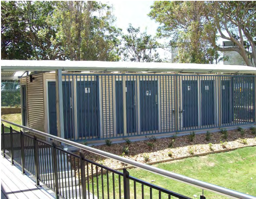
ABLUTIONS BLOCK, MOSMAN COUNCIL
